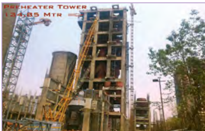
Preheater tower under mechanical erection at Manikgarh Cement Unit II, Gadchandur, Dist. Chandrapur, Maharashtra
