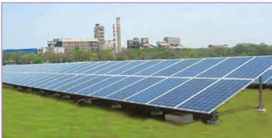
Solar photo voltaic power generation plant of 600 kw peak capacity at Century Cement, Baikunth, Dist. Raipur, Chhattisgarh
