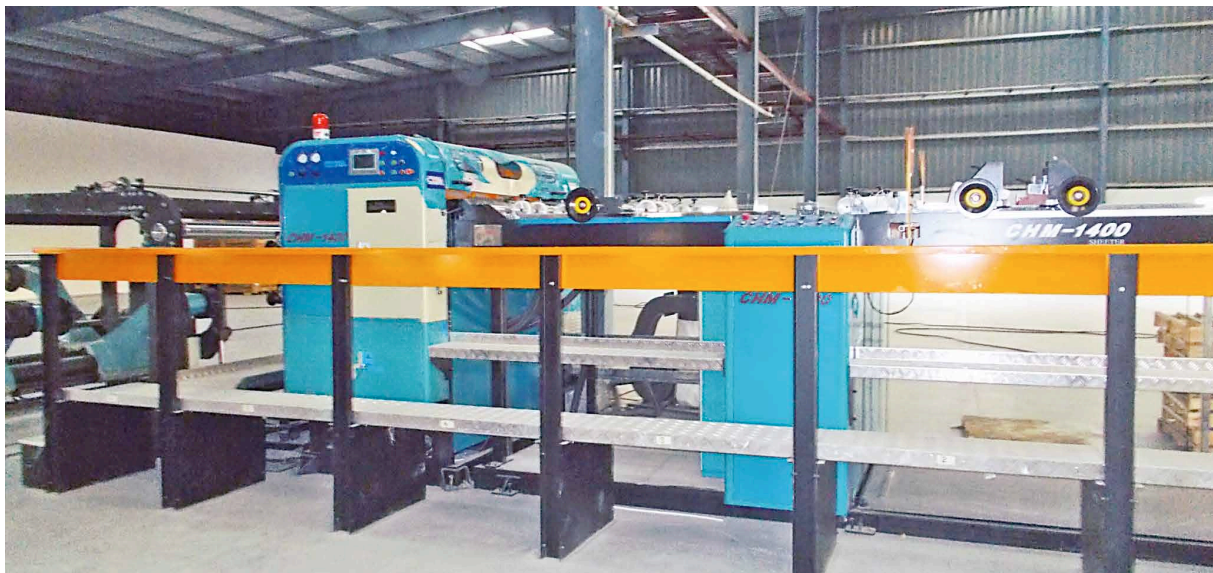
New plant at Bharuch, Gujarat of Century Pulp and Paper for cutting, finishing and packing of Board
