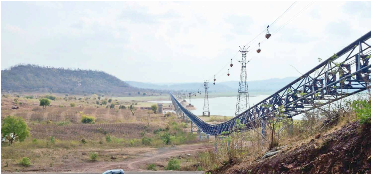
A View of single length Pipe Conveyor
