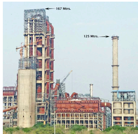
Manikgarh cement unit-II 2.8 Mtpa capacity under erection
